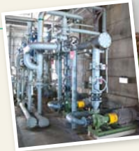
Water pump equipped with super high efficiency motors
