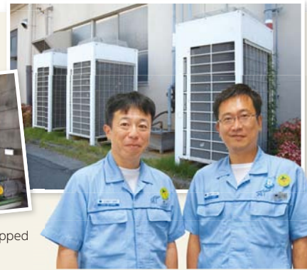
Air conditioner outdoor units coated with heat insulation paint
